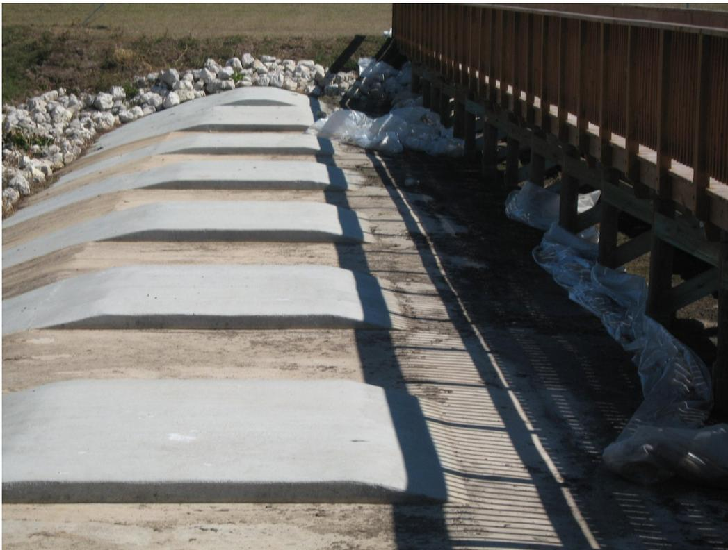
Figure 1-5. Outfall Weir Structure for the Wet Detention Pond.
