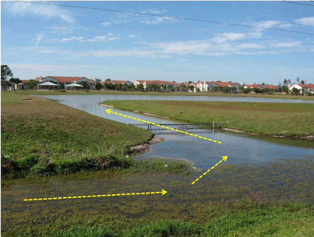
Figure 1-4. Diversion Canal into Wet Detention Pond.
